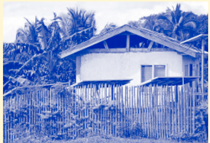
PV battery charging station at Malitbog (Photo: Approtech)
