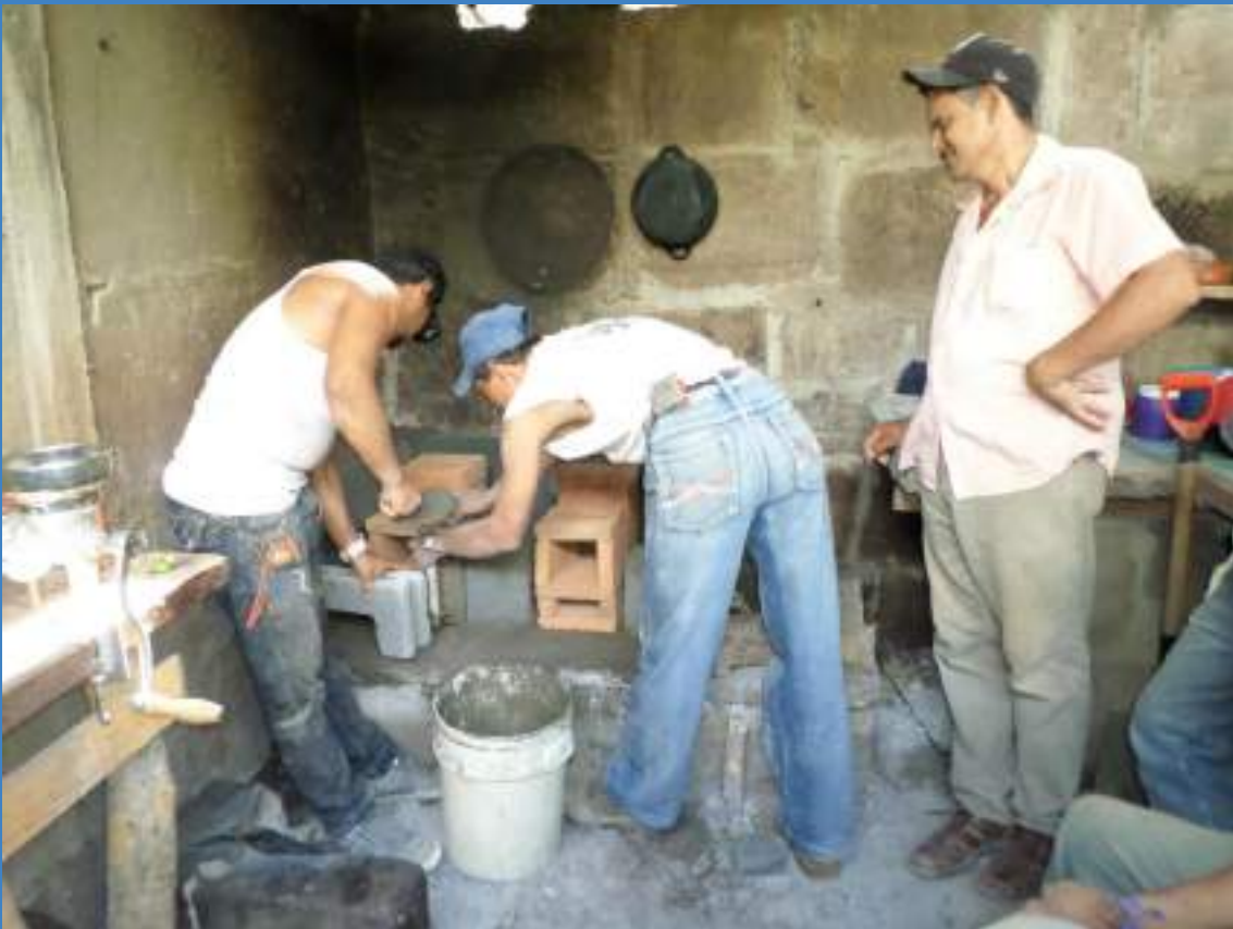
Stove construction in Sonzapote
