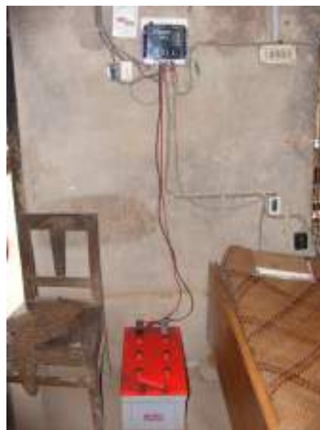
The SHS network without showing the solar panel on the roof and the lights. Note the charge controller at the center and the cellphone charger below on the right. Photo: David Hemson
