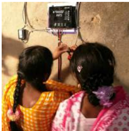
Trainees installing the charge controller. Women technicians report that they are not generally involved in home installations as this is regarded as heavy work. Photo: Grameen Shakti
