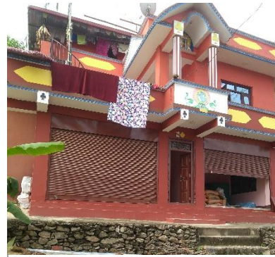
Photo 3: A well off house in Kavre
