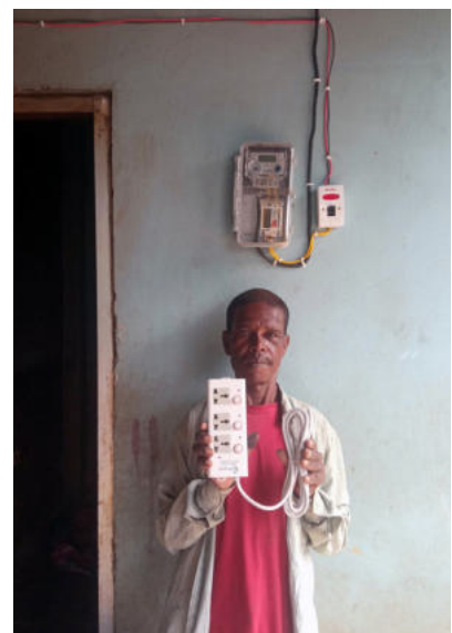
Wiring after upgradation
