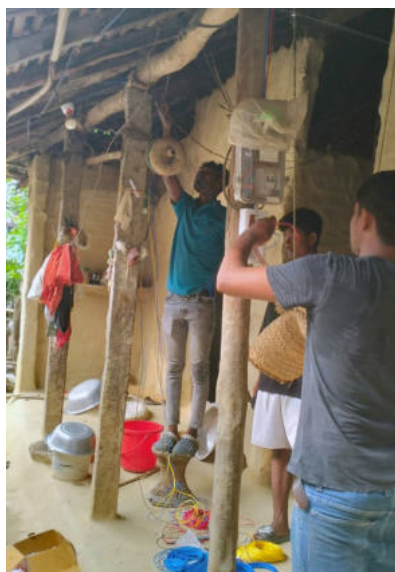
Wiring upgradation in progress
